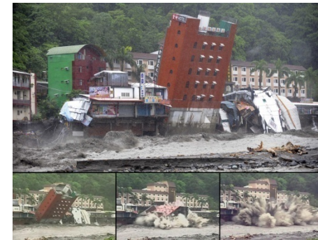
A hotel building fell into the river. (Taitung)
